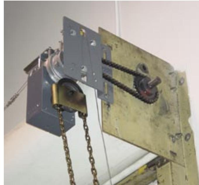
*After retrofitting, a fire door has a simplified self-contained system with a release and governor integrated into the retrofit fire door operator.*
