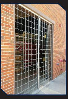
These gates are fabricated as horizontal and vertical rows of interconnected chain links in a square pattern suspended from a top track. With two different models, they can be used on truck bodies (specifically the cargo hold area of box trucks) and can also provide access control to buildings as well.
