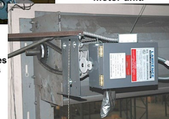
After retrofitting the fire door system is a simplified self contained system. Release mechanism and speed control governor are integrated into the motor unit.
